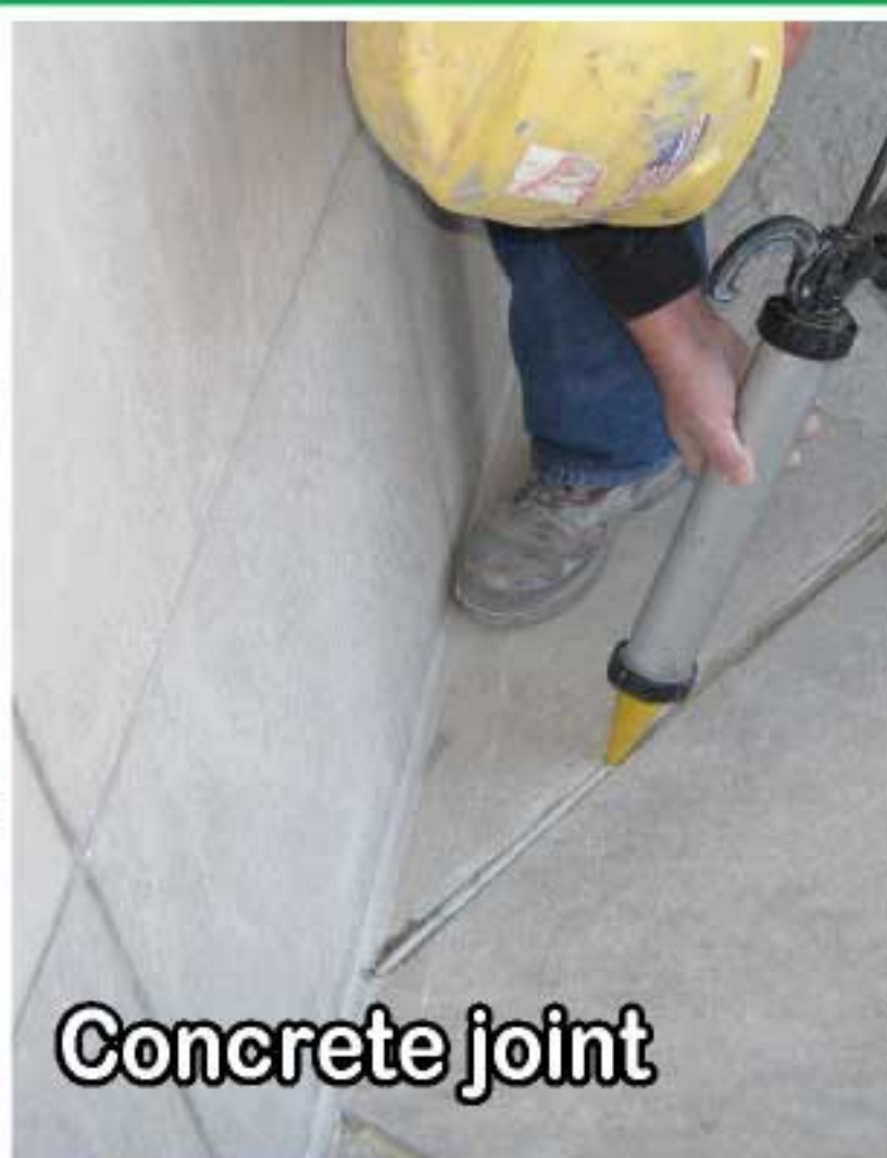
Precast wall panel joint
