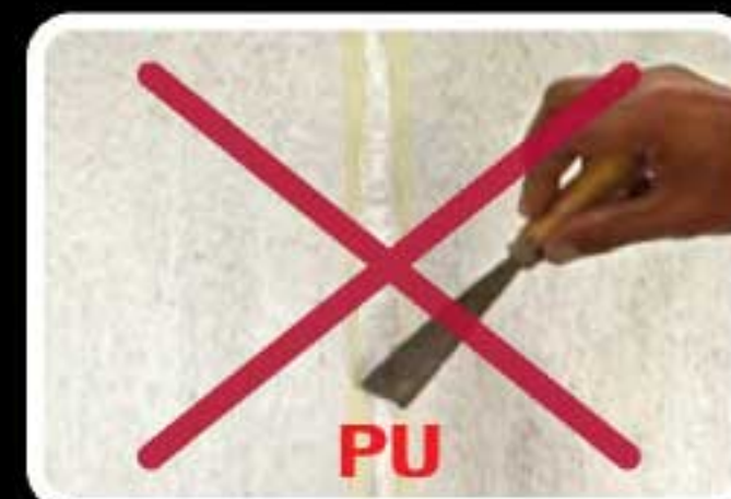
Difficult to tool (PU Sealant)
